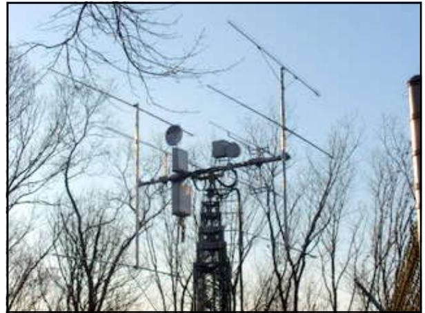
Outside there are motorized 106' crank-up towers. One for his 4 yagi 2m EME array and the other supports his terrestrial antennas from 6m through 24GHz. The microwave transverters are remotely mounted close to the loop yagis and dishes in weatherproof housings. There are bundles of control lines and coaxial cables up to the antennas. It is very clear that considerable time and effort was placed into the planning and construction of this installation.
